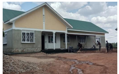
Progress so far
